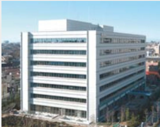
Ohi West Building
