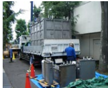
PCB waste being removed from the Ohi Plant
