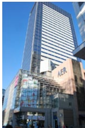
The AER Building where Nikon Plaza Sendai was opened
