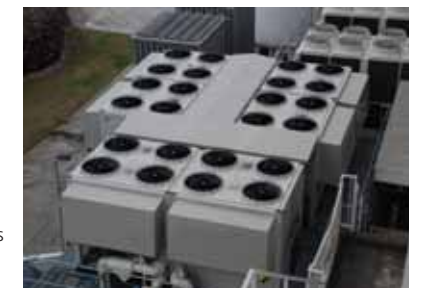
Heat pump chiller equipment of the steamless HVAC system (Tochigi Nikon Precision)
