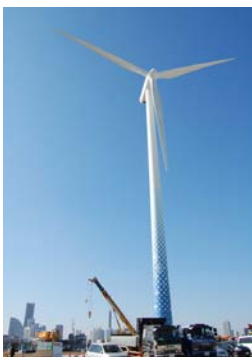
Wind Power Generation Facility in Yokohama City
