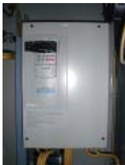
Pump inverter equipment introduced at the Mito Plant
