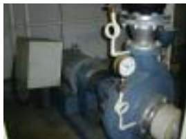
Pump inverter equipment introduced at the Mito Plant
